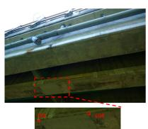
Figure 17. Damage at the bottom of the main beam at the test site: Refilled concrete.
